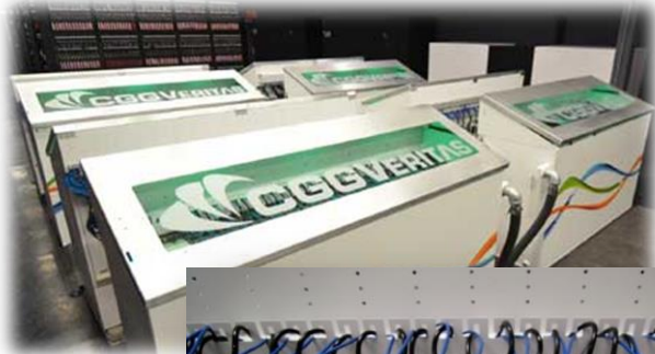
“Submerged Supermicro Servers Accelerated by GPUs”
